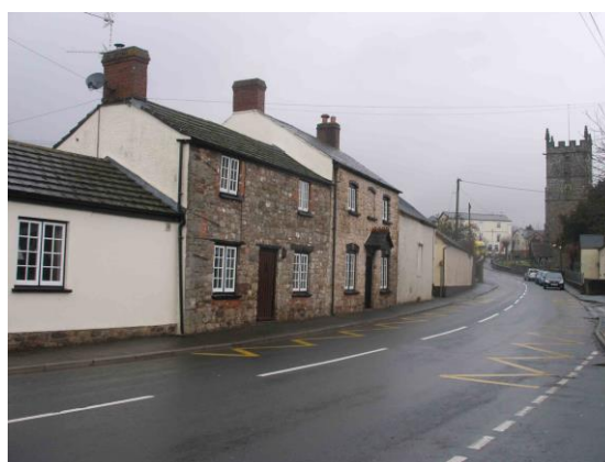
Fig. 55 Elm Cottages , also on the Chepstow Road, are more vernacular in character but have regularly proportioned front elevations in rubble walls. The Beaufort Arms and the tower of St Cadoc's church are in the background.
