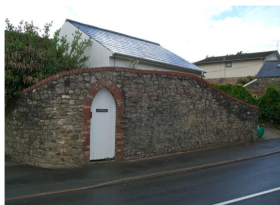
Fig.30 Red brick arched doorway set in the stone walls on Chepstow Road
