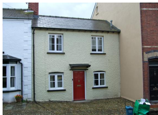
Fig.62 No.7 Castle Street displays typical features prevalent in Raglan, with rendered roughcast walls, slate roof, casement windows and stone setts or cobbles to forecourts
