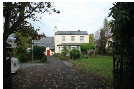
Fig.68 Orchard Lea makes a positive contribution to the conservation area
