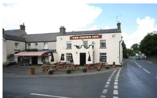
Fig.44 The Crown Inn, a prominent building set on a key corner in townscape terms
