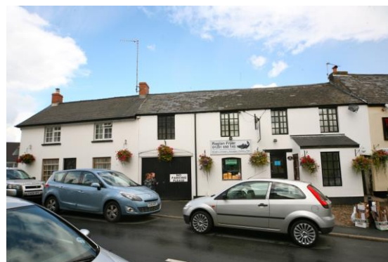
Fig.39 White painted rendered buildings with natural slate roofs predominate the High Street
