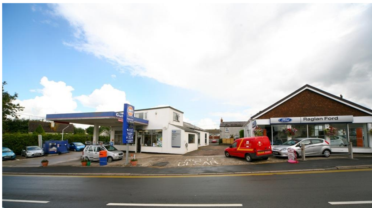
Fig.33 The garage forecourt disrupts the traditional street scene, breaking down the townscape on the north side of the High Street
