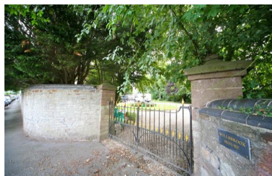
Fig.45 Grand entrance into Willsbrook House with rubblestone walls topped with engineering bricks
