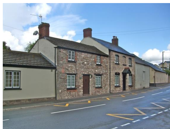
Fig.25 Elm Cottages, Elmcote and attached barn on Chepstow Road form a group making a positive contribution to the character and appearance of the conservation area
