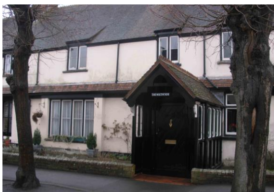
Fig. 58 The Malthouse in the same terrace is distinguished by an unusual timber passage porch. The terrace is also unusual in having a continuous pentice roof to the ground floor
