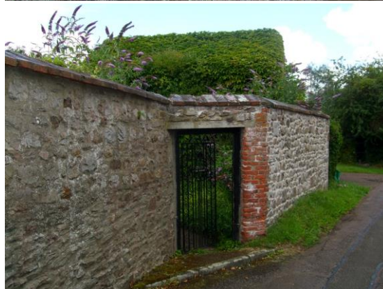
Fig.63 Stretches of rubblestone walling with brick cappings, along Primrose Lane
