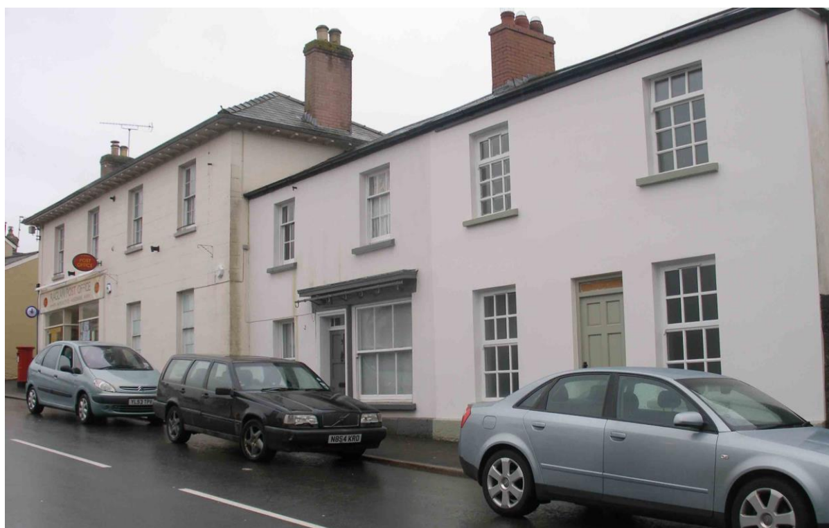
Fig. 52 Raglan House (to the left) dating from the early 19 th century in the centre of the High Street has typical late classical features such as a low hipped roof with bracketed eaves. The shop front is a later addition.
