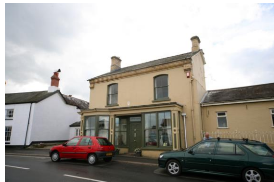
Fig.36 Two traditional shopfronts on the High Street at Extons & London House
