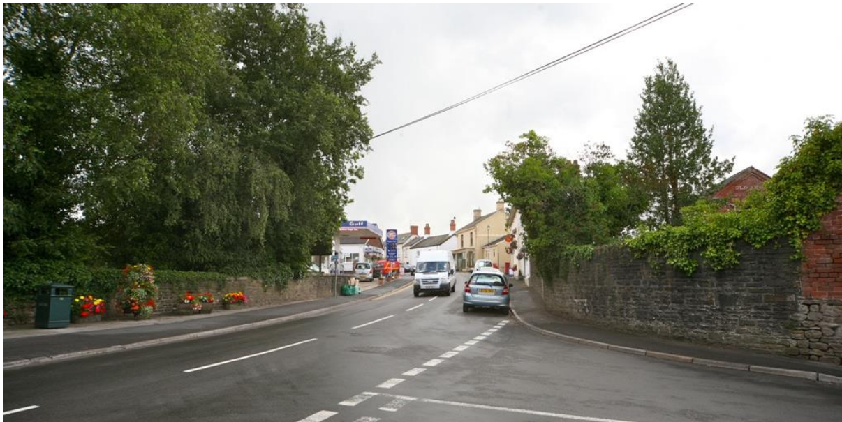
Fig.47 View east to the High Street, well-defined by built form along its length
