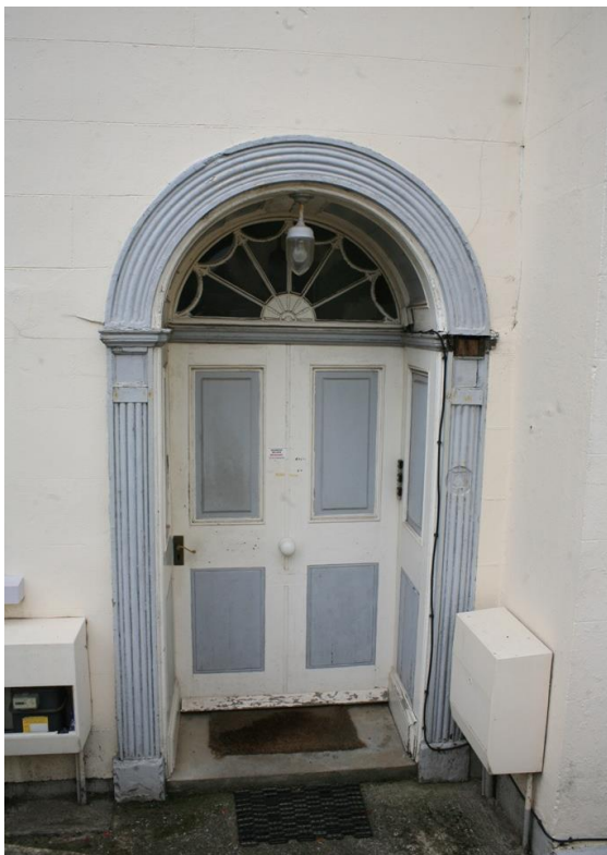
Fig.35 The fine classical doorcase at Raglan House
