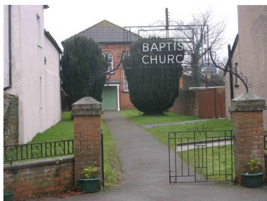
Fig. 56 The Baptist Church set well back from Usk Road, has the simple 'stripped' neo-classical characteristics of a mid 19 th century non-conformist chapel.
